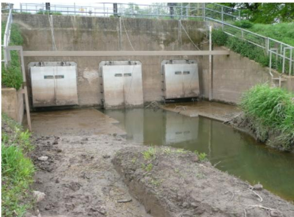
**Fig 1: Typical flood defence doors/flaps.**
